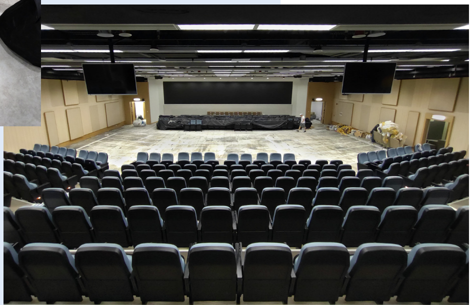
Lecture room 1 at the Yasumoto International Academic Park during construction
